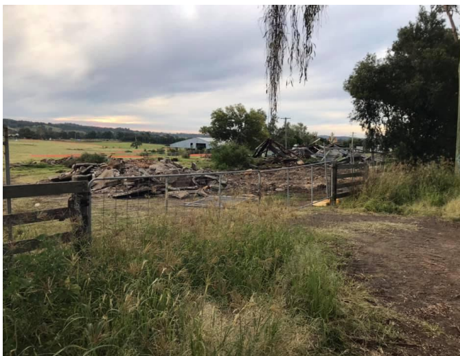
Demolished farm shed in Stevens Road
